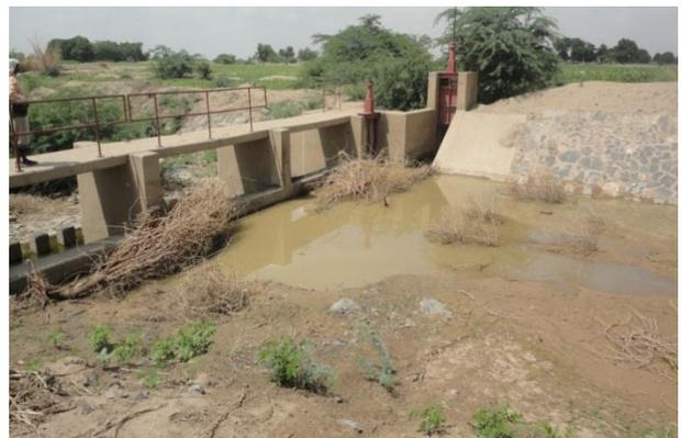
Figure 3. A sample of blocked irrigation Channel
